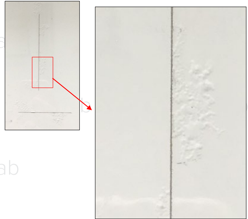
Corrosion morphology – Type B
